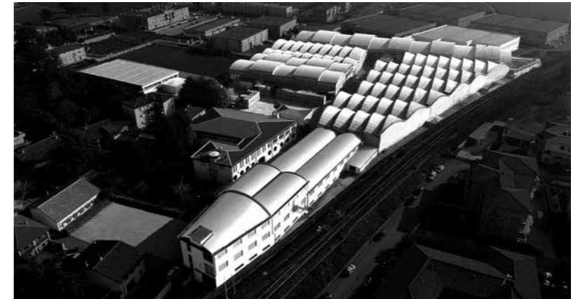
SCAB sede/headquarters - Coccaglio (BS) Italy
